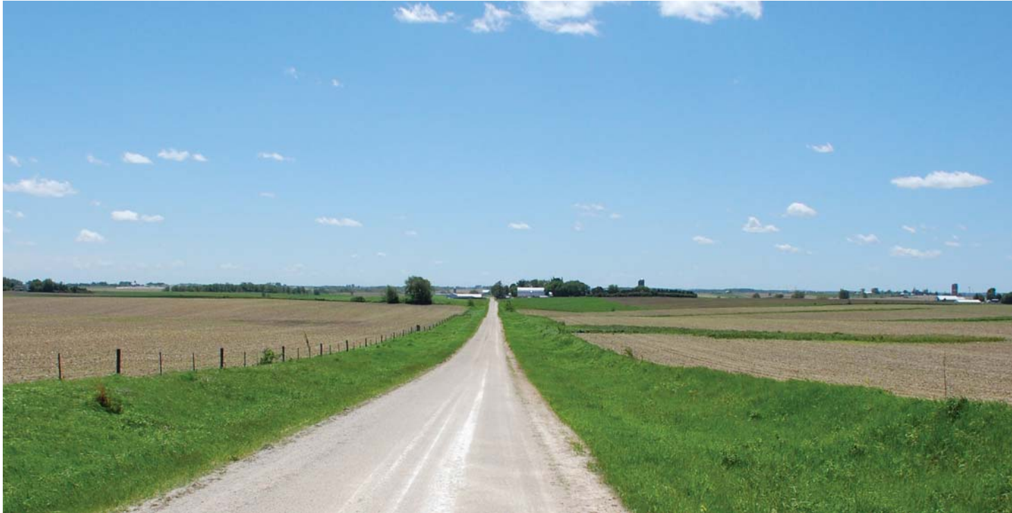
Right-of-Way Width: 60 feet Location: 381st Avenue, Minnesota
